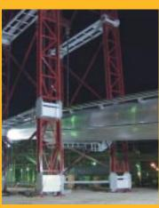
The MLT competed successfully against several heavy lift cranes. The MLT does not congest a job site like a large crane allowing other work to continue. This alternative heavy lift system is a versatile piece of equipment that is customized to each specific project and typically has lower ground loading and higher safety margins than comparable heavy lift cranes. Hats off to Barnhart engineers and the crew for safely making Barnhart history.
