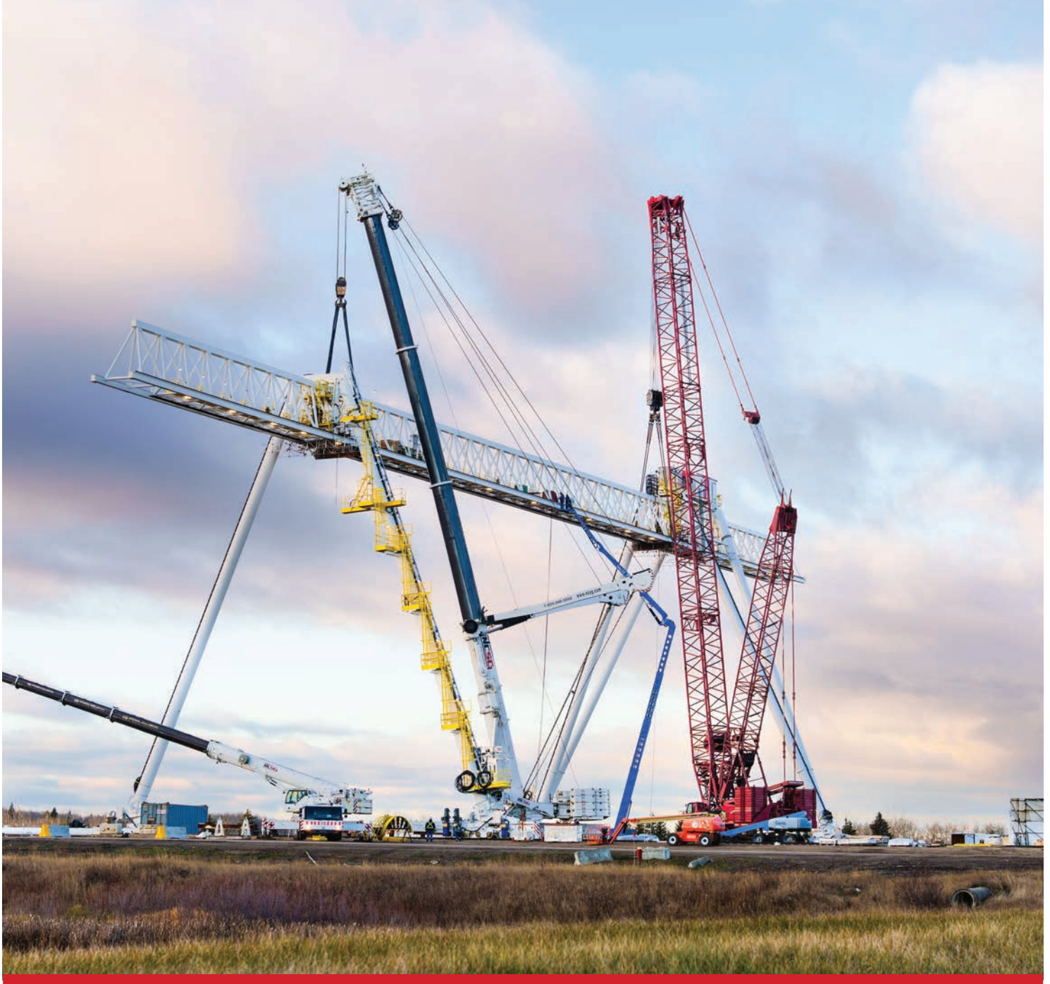
Edmonton's Manitowoc M18000 and Liebherr LTM 11200 tackled critical crane work at a pulp mill.
