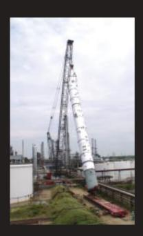
In August, Barnhart performed roll off operations, on site transportation and the heavy lifting of a 150 ton splitter column and a 100 ton reactor for a Texas
