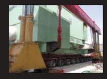
Once in Jamaica, the boiler was rolled off the barge with platform trailer, hauled 15 miles in 4 hours (220 overhead lines had to be relocated). Barnhart then set the boiler on its foundation with a gantry system. The project was completed on time and without incident.
