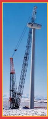
Barnhart Crane was contracted by a major wind turbine manufacturer to perform all logistics and erection aspects of an extremely aggressive wind project in Wyoming. The project was awarded on the basis that Barnhart could safely and efficiently transport and erect 80 1.8 Megawatt machines on 65 meter towers in less than 3 months.
