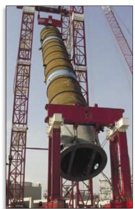
Barnhart's proprietary Modular Lift Tower (MLT) erected a 650 ton reactor in support of a Clean Fuels Program at a Detroit refinery. The 130' long reactor was rolled off a barge with 36 lines of platform trailer and transported to the MLT. A pair of 450 ton strand jacks handled the main lifting while tailing operations were executed with the Modular Tailing Tower (MTT) in lieu of a large tail crane. In four hours, the reactor was vertical and safely on the anchor bolts.
