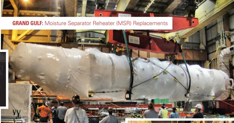
arnhart replaced two MSRs in the turbine building via a passage through a bio shield wall on the turbine deck. Barnhart's standard jack and slide methods were used along with custom-fabricated saddles to remove the components. The team also used a specialized rotating lifting beam and two 250-ton overhead cranes in tandem configuration.
