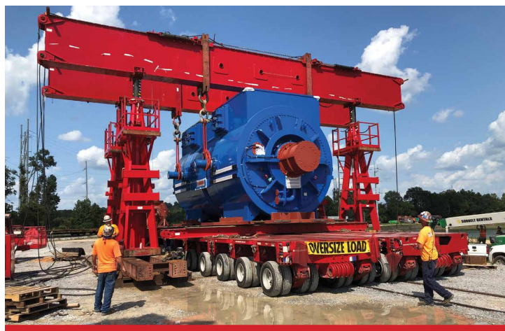
Barnhart workers offload and haul a 725,000-pound steam turbine generator using 500-ton one-shot gantries.
