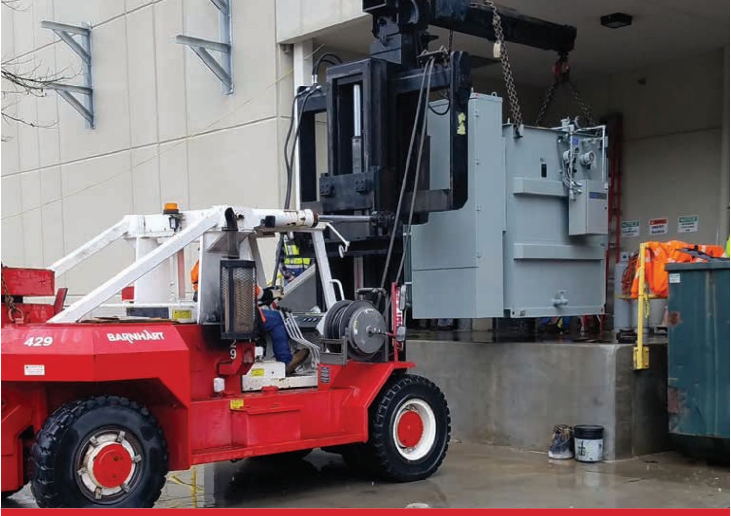
A Barnhart operator uses an 80K Taylor forklift with a boom attachment to set a transformer at a research lab.
