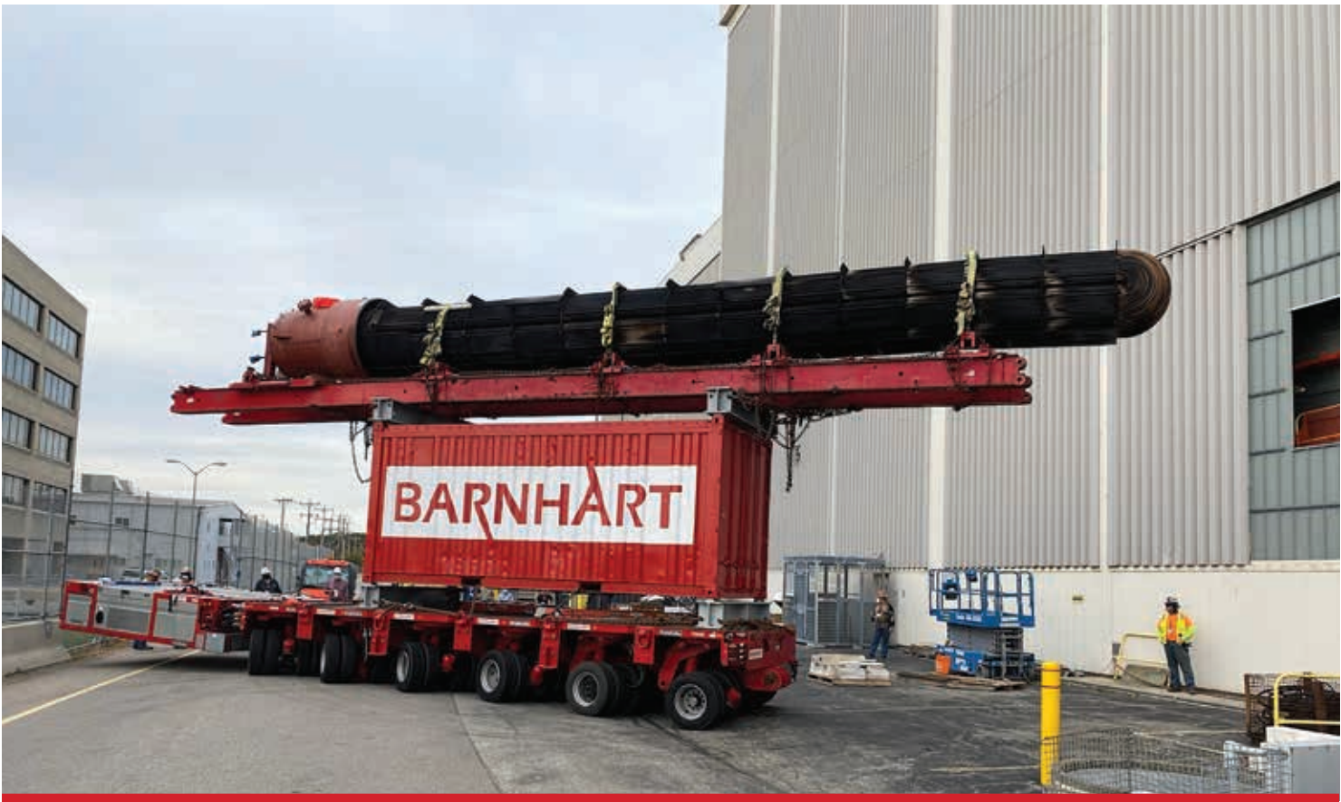
Two 40' long feedwater bundles were removed and replaced by the Middletown team during a planned outage at a nuclear plant in Connecticut.
