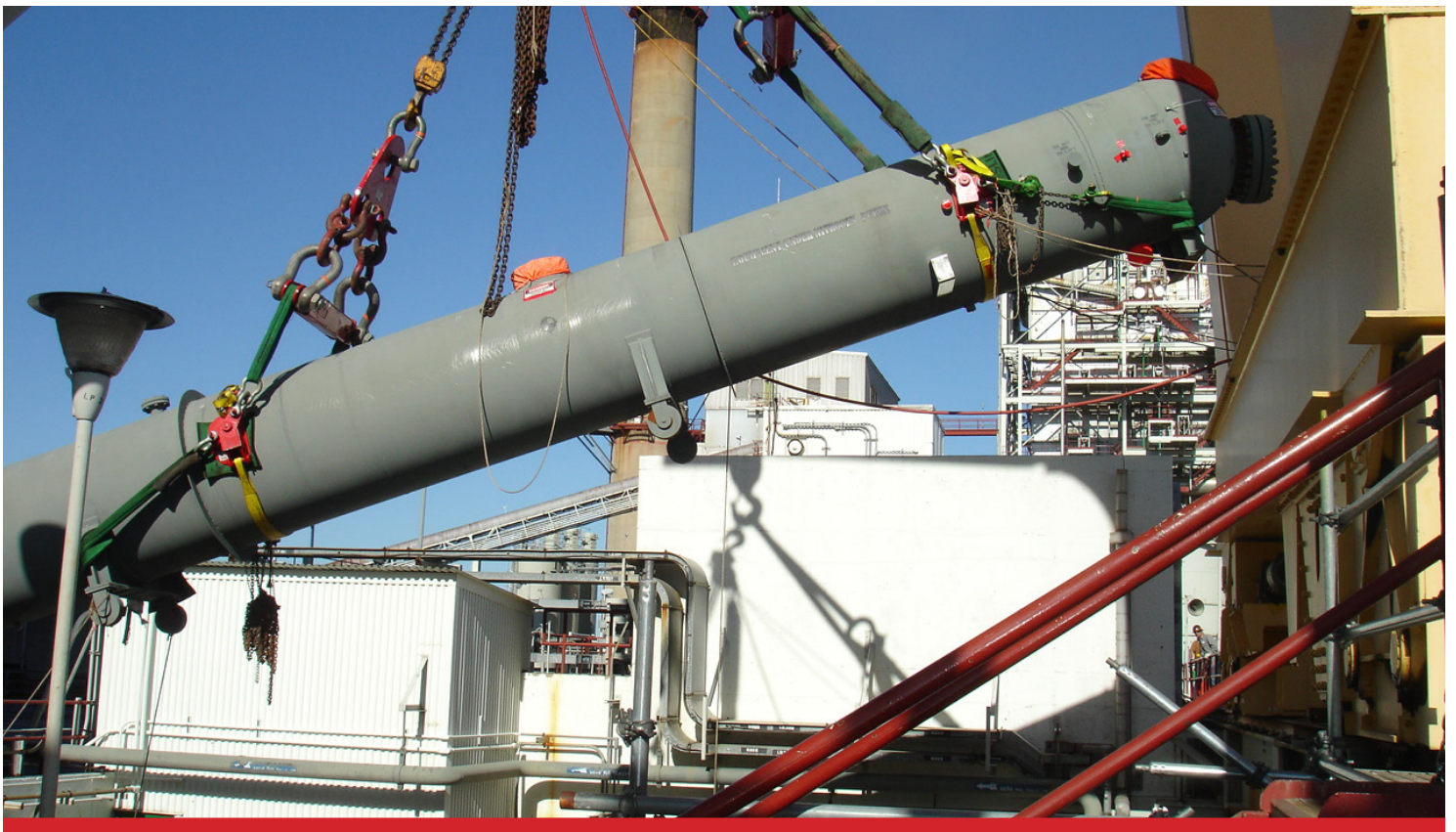
Temporary trunnions allow for rigging attachment points at specific locations along the length of the vessel.
