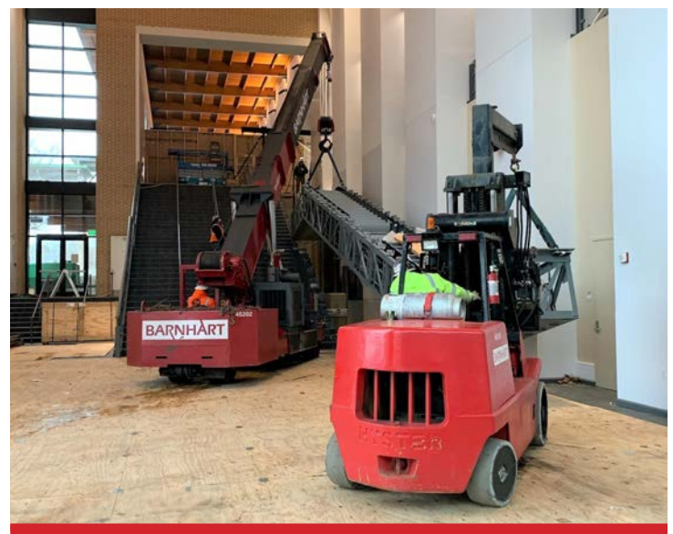
5 Plus, the project was completed in less than two eight-hour workdays.
