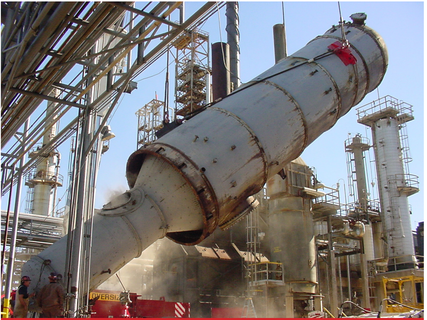
Trunnions help protect the shell of the vessel during the upending process.
