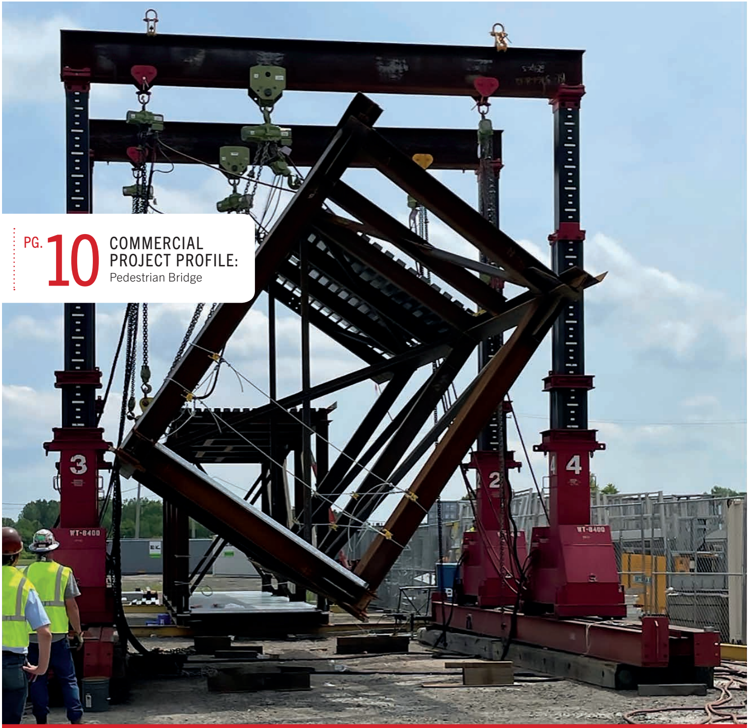
Barnhart staging a pedestrian bridge section at its yard.
