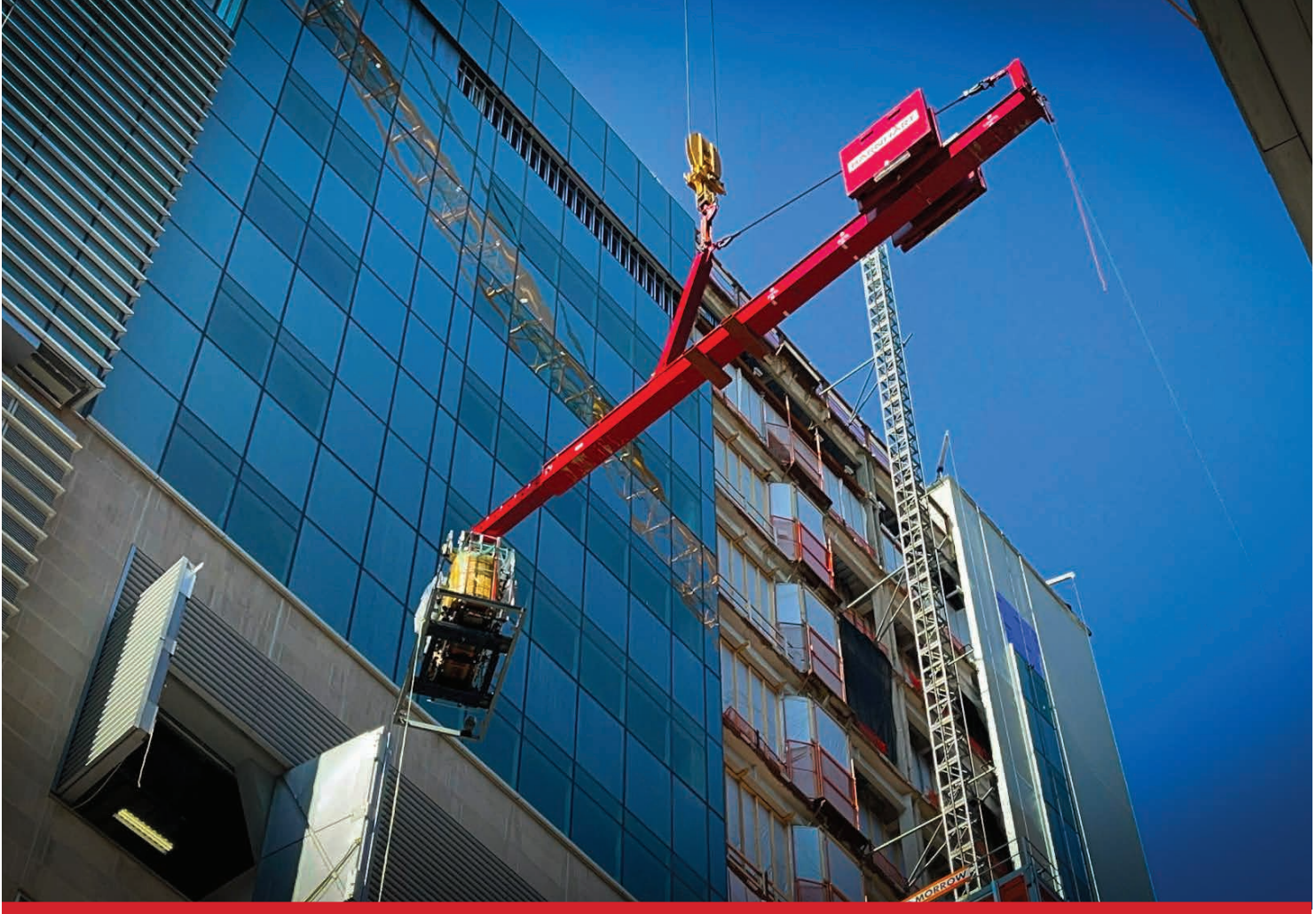
St. Louis used its Movable Counterweight Cantilever System (MOCCs) to install new transformers in downtown St. Louis.
