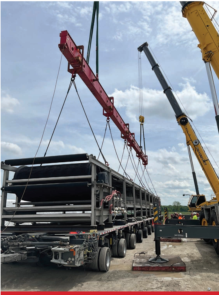
The Madison team prepares to lift a horizontal belt filter at a power plant using two telescopic cranes.
