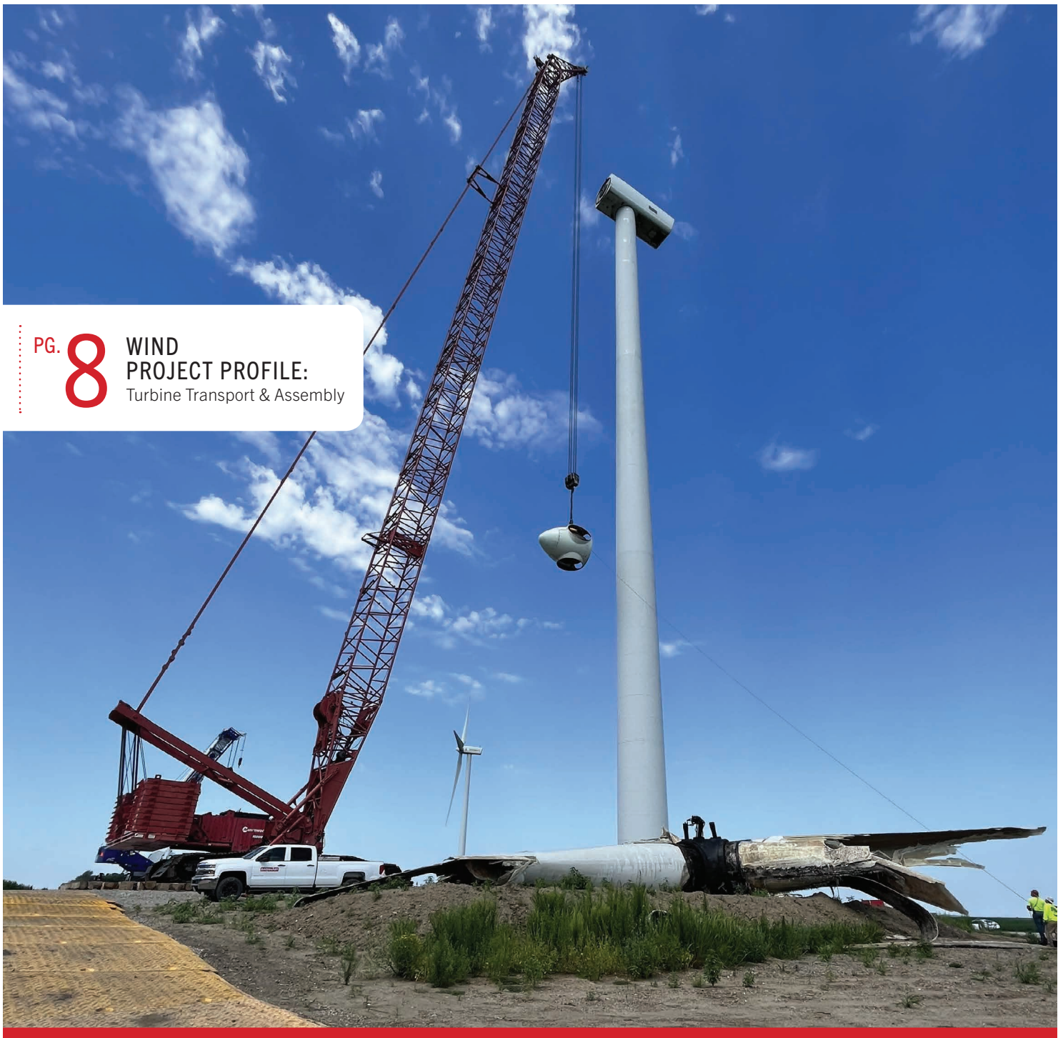
Barnhart at a project to replace burned out turbines with new ones.
