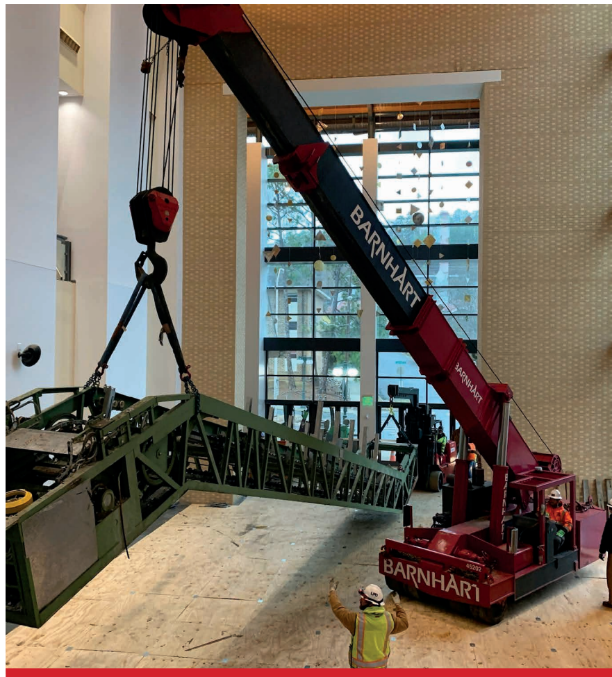
The Little Rock branch at the Hot Springs Convention Center removing and replacing an escalator using a Mobi-Lift and 18K forklift.
