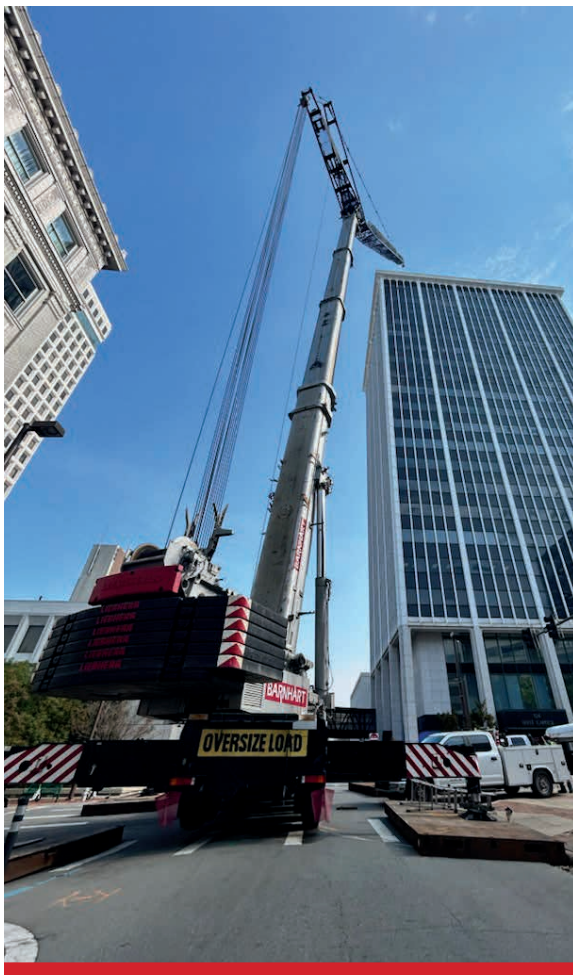
The crew working at 280' elevation servicing rooftop chillers with a 600-ton crane in downtown Little Rock.
