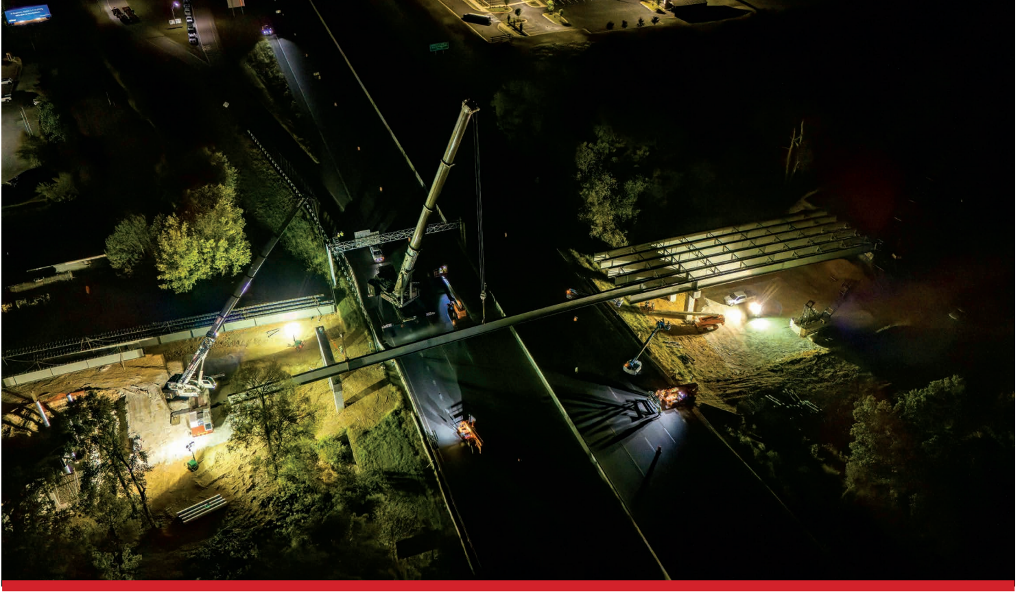
The Springdale branch setting bridge girders at night handling weights of up to 126,000 pounds per beam and lengths of up to 230'6".
